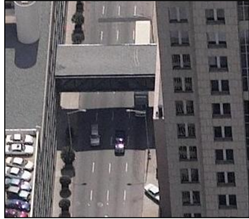
Figure 4: Raised Pedestrian Crosswalk
